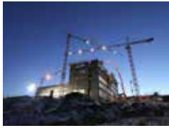
CANTIERE WORK SITE
